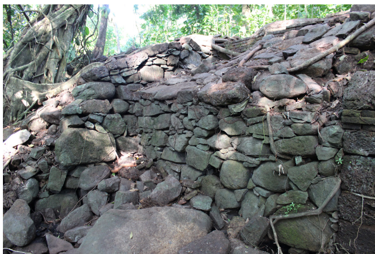
Figure 4 Glacis de moellons
